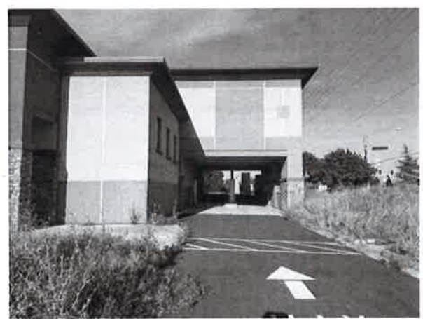
1 VIEW OF EXISTING DRIVE THRU
