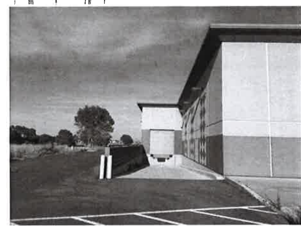
VIEW OF EXISTING LOADING DOCK
