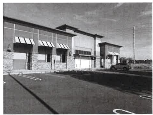
2 VIEW OF EXISTING ACCESSIBLE STALLS
